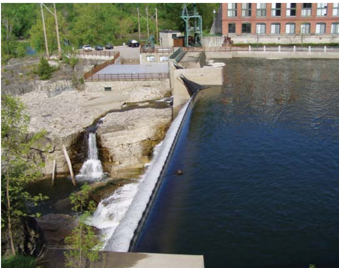
Winooski Hydropower from above the dam
